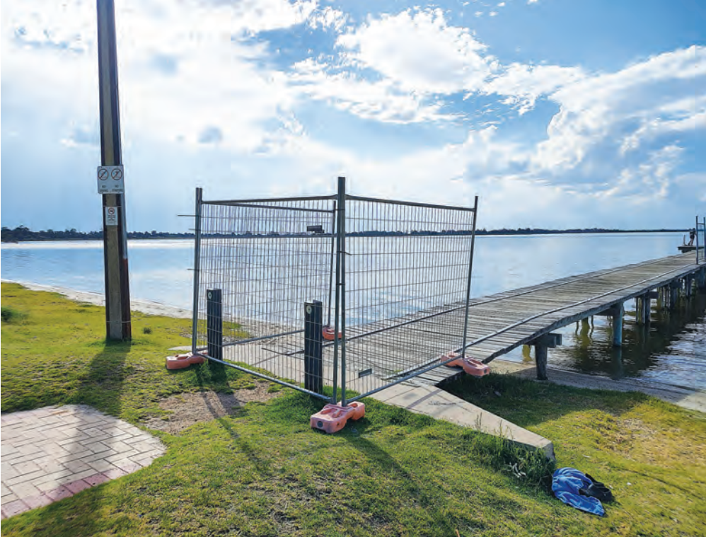
The Lake Bonney Jetty is to be closed until further notice due to vandalism. PHOTO: Sebastian Calderon
